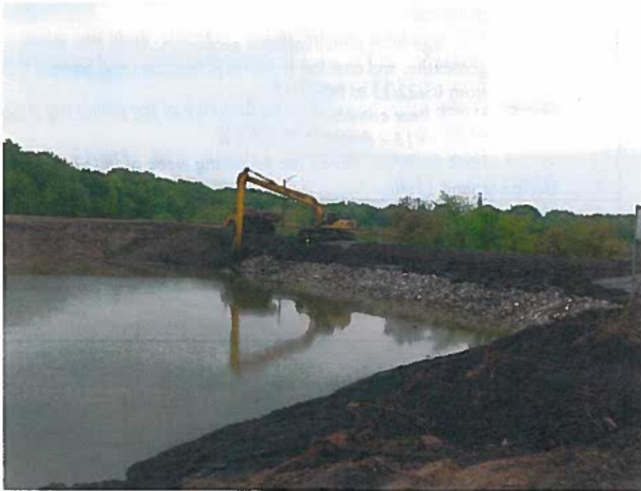
Northeastern view of slope stabilization layer construction along eastern slope
