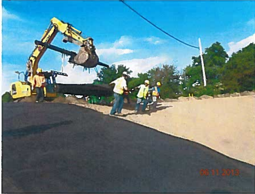
CAAW begins deployment of geotextile
