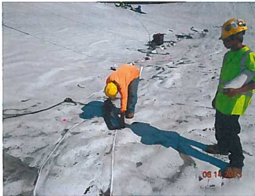
Vacuum testing on extrusion welds
