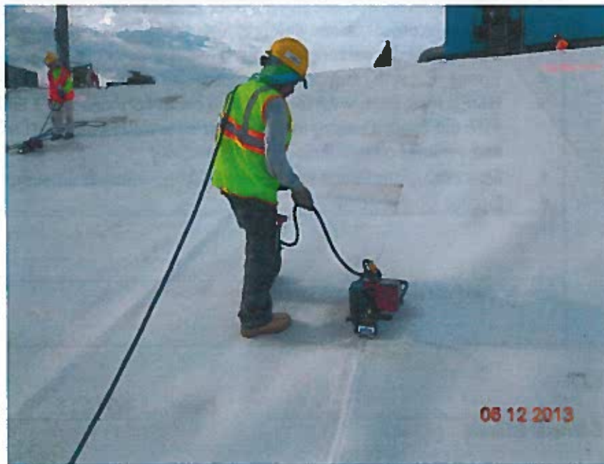
Fusion welding HDPE panel seams (looking south)
