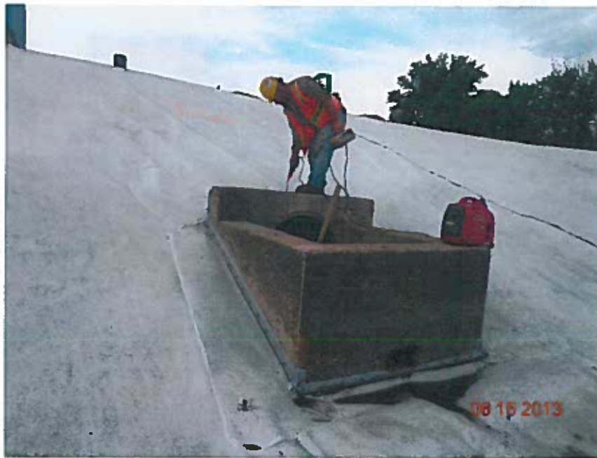
Spark testing on extrusion welds at structure (looking southwest)
