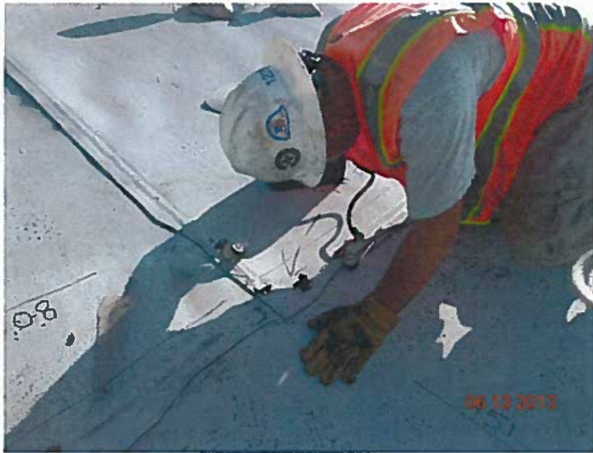
Non-destructive air testing of fusion welds
