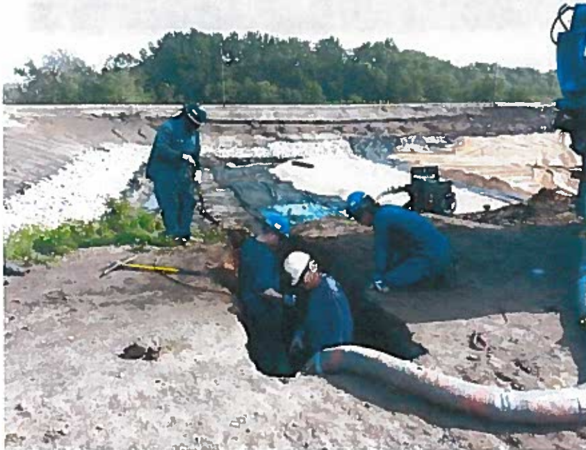
View of ongoing trench vacuum excavation for side-chute
