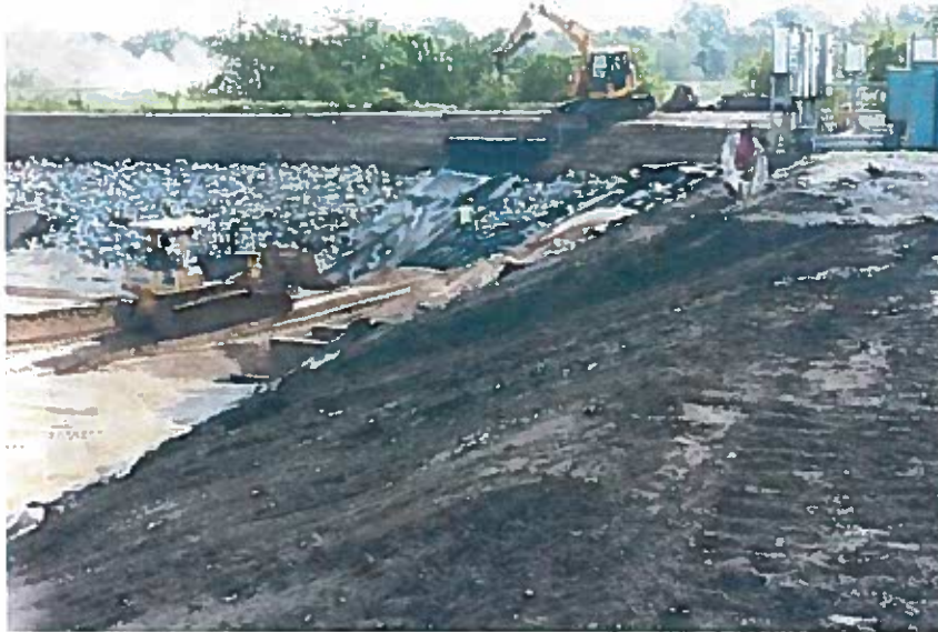
View of geotextile placement above riprap stabilization layer on eastern slope
