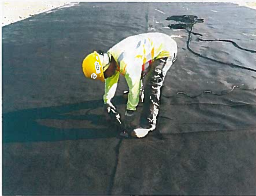
Heat bonding the geotextile panel seams
