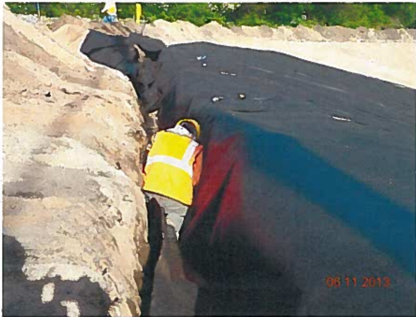
CAAW placing geotextile in the anchor trench
