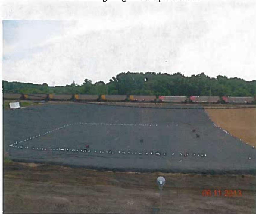
Northern view of placed geotextile at end of day
