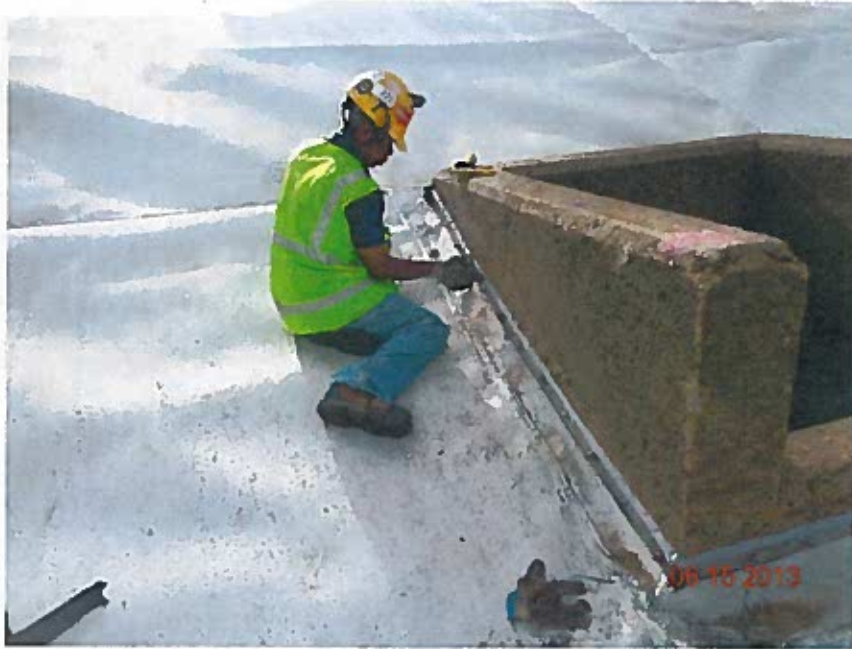
Batten strip attachment to structure (looking southeast)
