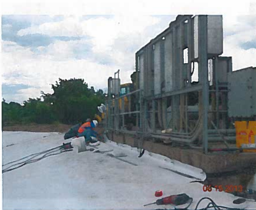
Batten strip attachment to pump pad structure (looking southeast)
