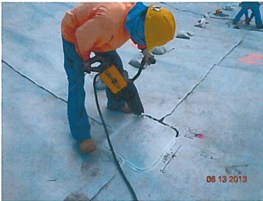
Extrusion welding patch over a repair location
