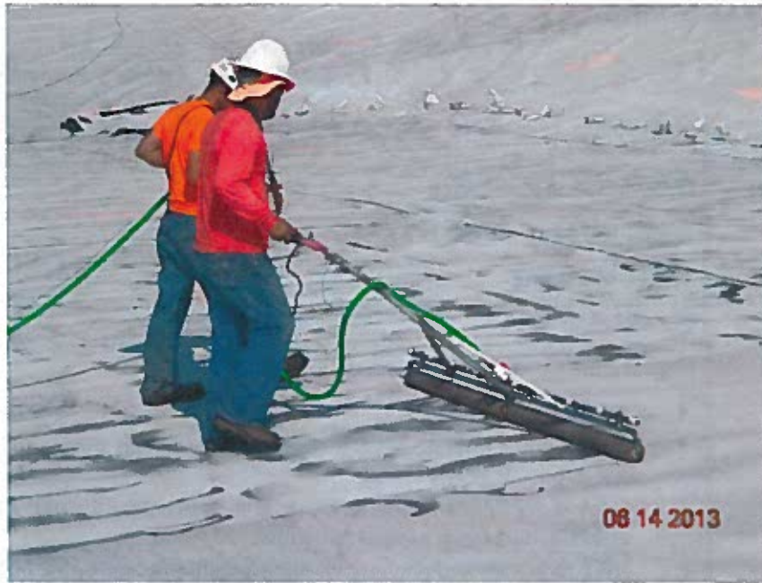
Leak location survey along bottom of basin
