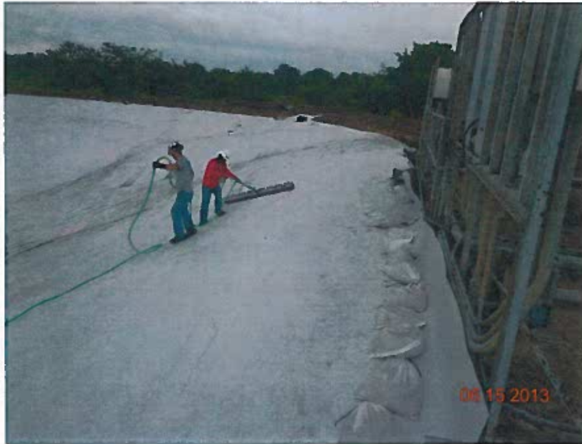
Leak location test being performed on basin slopes (looking east)
