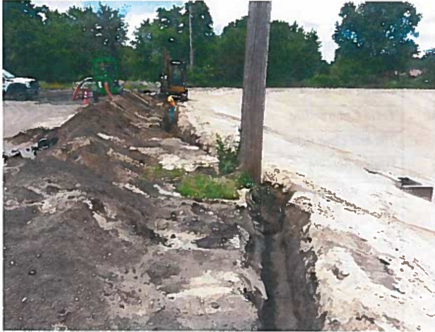
Western view of anchor trench excavation on top of south slope
