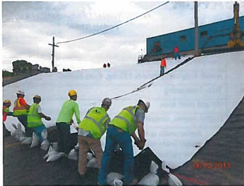
Deployment of HDPE liner on southern slope (looking southeast)
